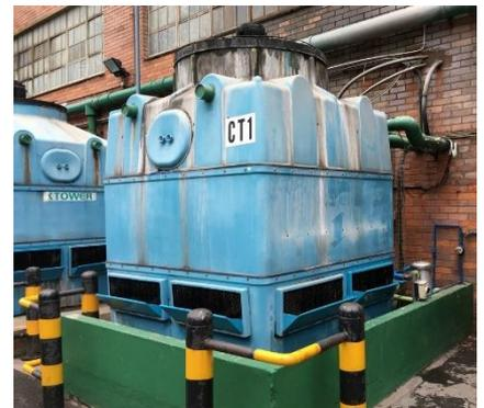
So far the main focus has been to evaluate the approach between water and wet bulb. But there is much more to it. It becomes obvious that the M&V for the cooling towers can be improved. More can be done to create not only energy efficiency and benchmarking but also define the "water efficiency" of the tower. ClimaCheck is in the process of initiating field tests with the new cooling tower evaluation algorithms on several markets. Contact us if you have cooling towers in
